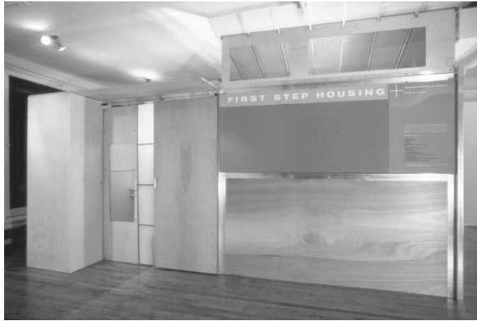
First-Step Housing, Van Alen Institute, Fall 2000. View of two attached units oriented at 180 degrees. Three sliding panels of interchangeable position and function and varying degrees of transparency compose the front wall. They are set back from the exterior edge of the closet to create a zone of transition and identity like a porch.
