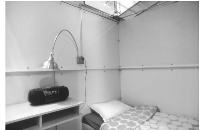
Common Ground's brief requested single rooms for single men, but we conceived a system capable of different occupancies and configurations. The units can be combined to have multiple bedrooms or shared and contiguous living arrangements.
